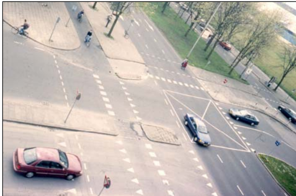
Large intersection with multiple crossings - note three sets of saw-tooth markings: one for pedestrians, one for cyclists, and one for vehicles.
